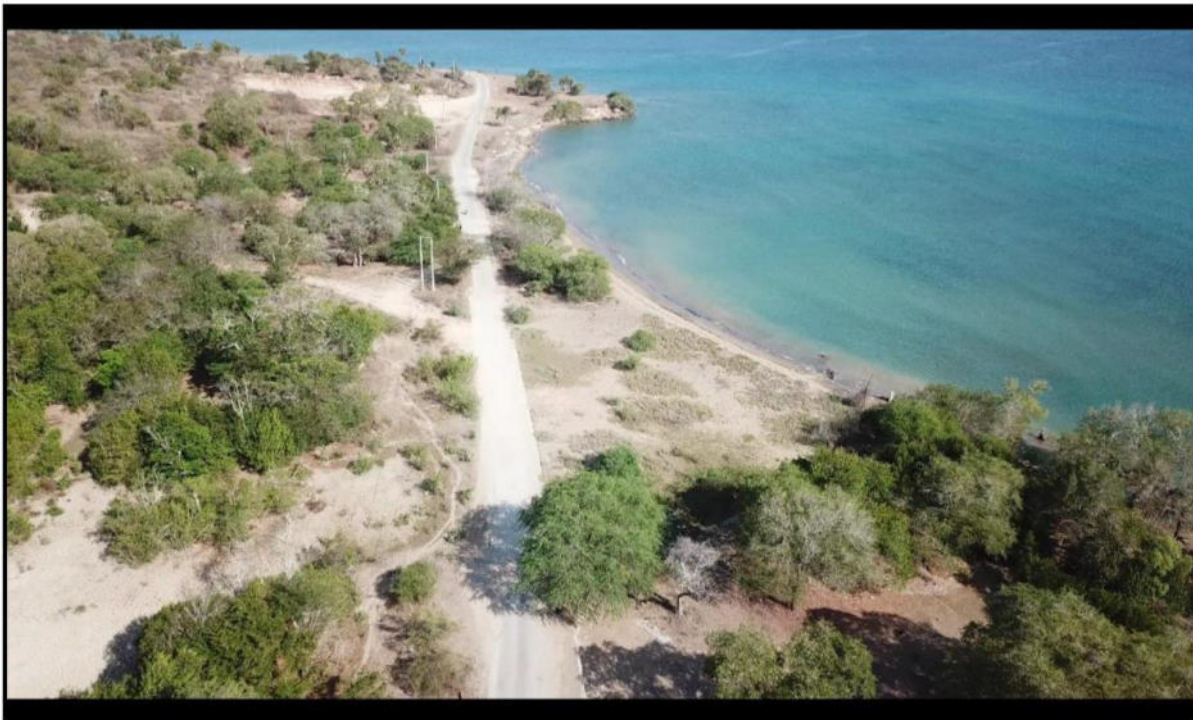
Malailada Causeway towards West end (aerial photo looking east to west 2021)
